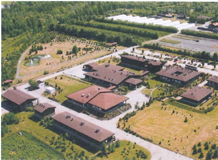
Above: Aerial view of FGB
